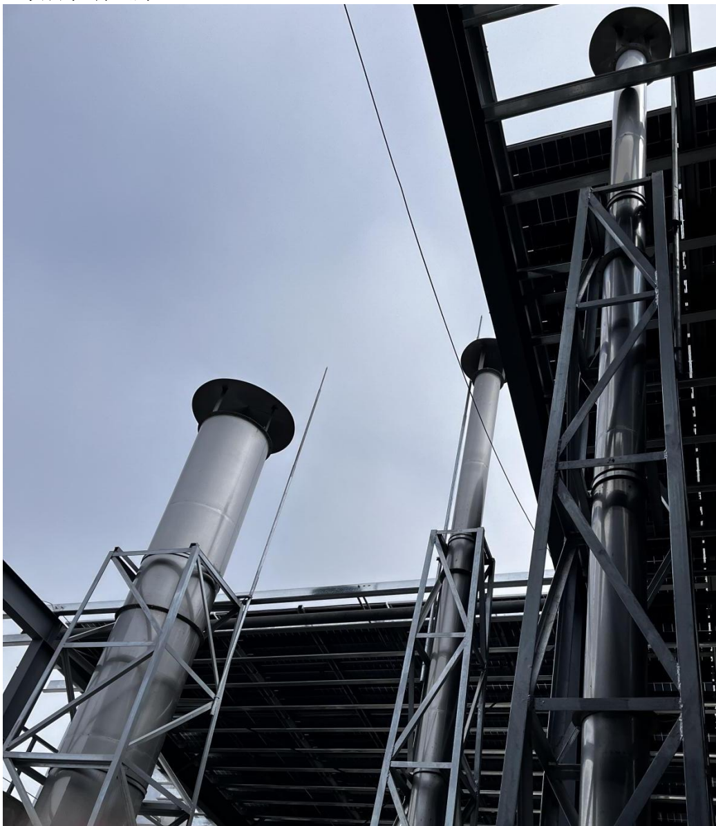
舟皿喷砂粉尘、产品喷砂粉尘、切割粉尘排气筒
